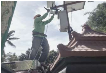
Figure 1. Installation of evacuation guidance instrument. Photo by: MRC
